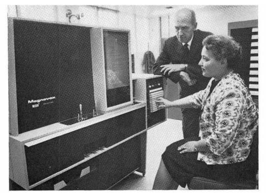
RETRIEVAL/READING MACHINE in Central Technical Files is demonstrated by Betty Baros. Selection is made by keyboard, and 180-200 film chips in each capsule are scanned until desired one is located. An item can be located in an average of eight seconds. Clarence Schooley of Records Management Division helped train Betty.
